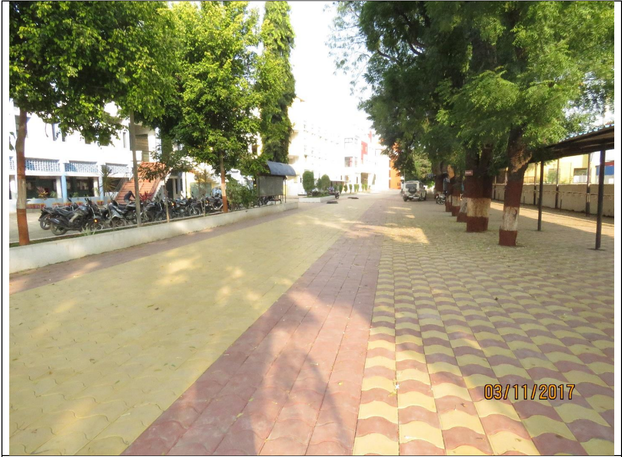
Entrance and Parking
