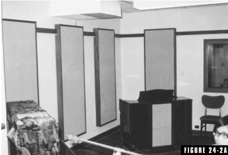
(A). The simplest and cheapest way to adjust the reverberation characteristics of a room is to use removable panels. These photographs were taken in the studios of the Far East Broadcasting Company, Hong Kong.
